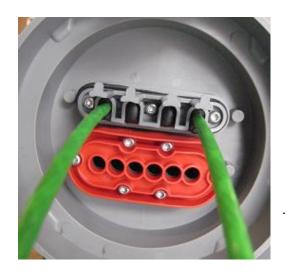
8. If a black edge of rubber is visible around the Window Cut port seal, the seal is made correctly.
