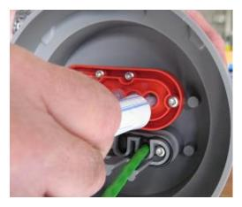
13. Cut the outer sleeve of the cable / duct perpendicularly. There must not be any lengthways cuts past the end.
