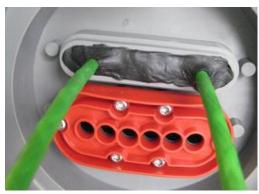
6. Roll the long piece of sealing rubber into the shape of a sausage and divide it equally into the port.
