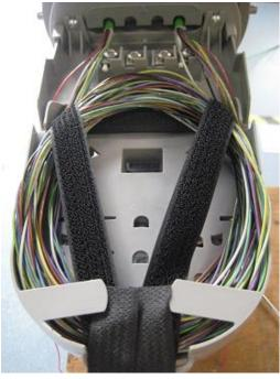
9. Place the overlength of the tubes / fibers that are not being used under the velcro
